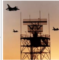
Air Traffic Radar
